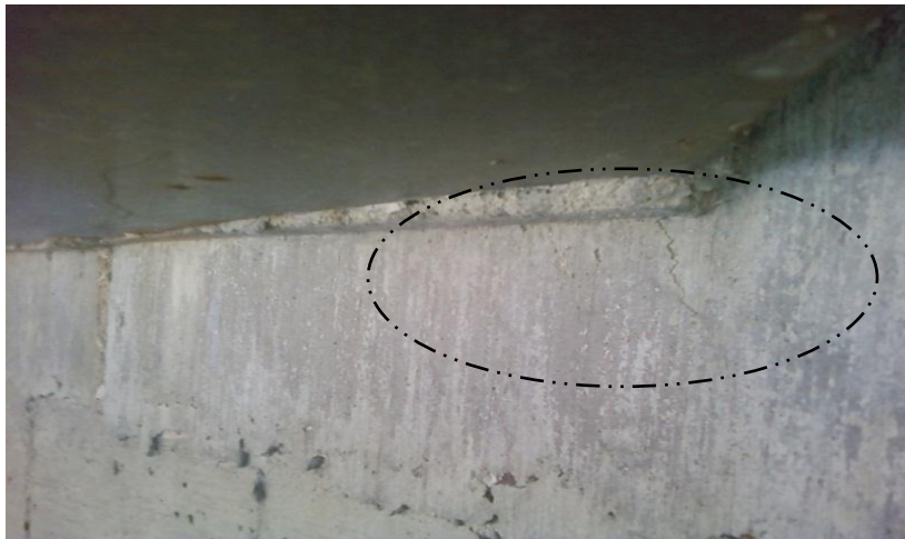
Figure 4.2. North Abutment and Bottom Flange Interface
