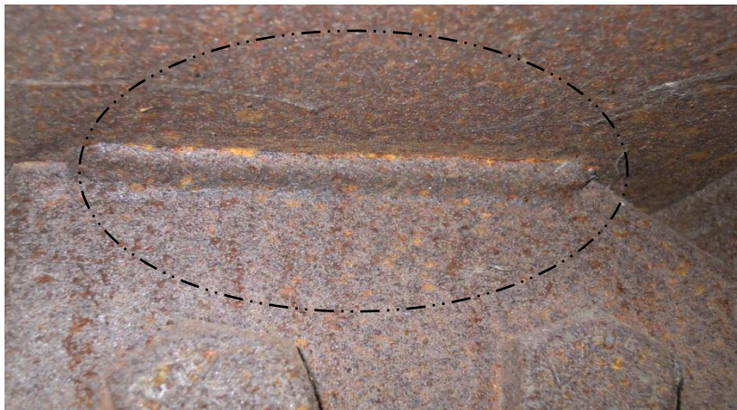
Figure 4.9. Girder-to-Diaphragm Welded Connection
