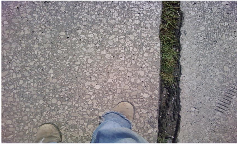
Figure 4.6. Approach Slab/Bridge Joint
